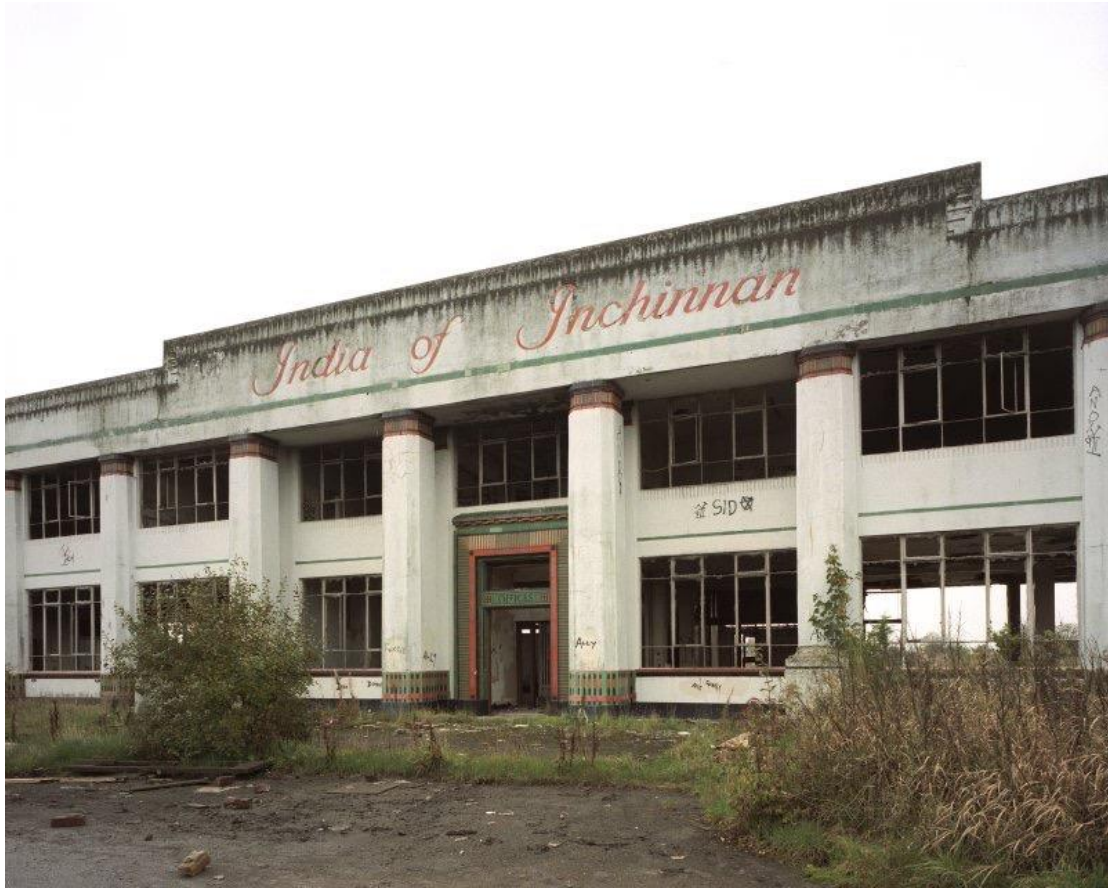
Façade of India of Inchinnan prior to renovation.
