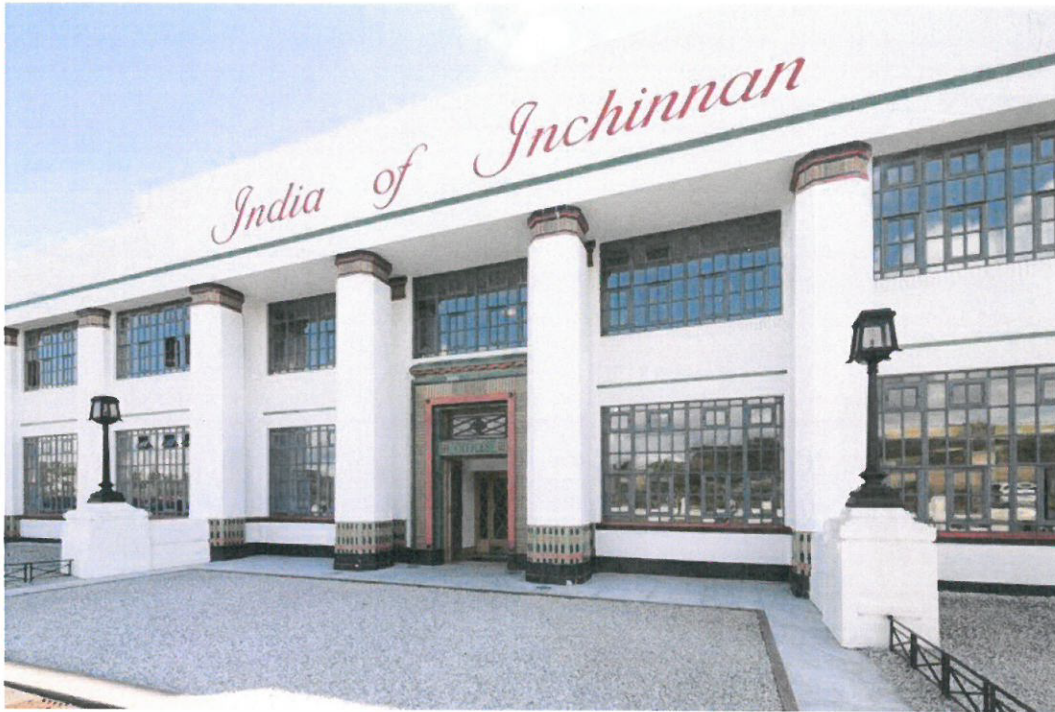
India of Inchinnan after renovation.
